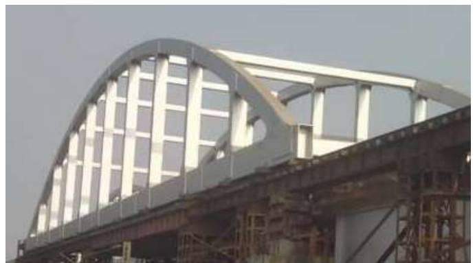
Bow String Girder - 60M Span
