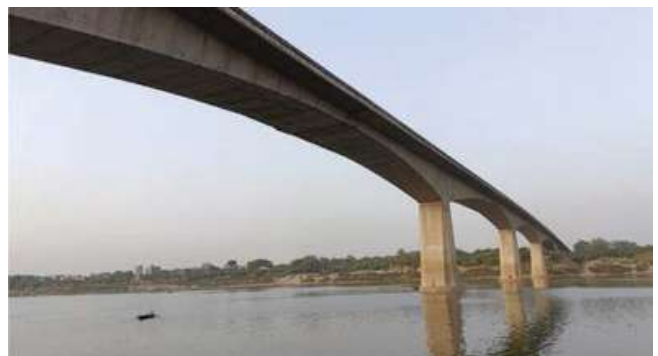
Vishwasundari Bridge Uttar Pradesh (Repair and Rehabilitation)
